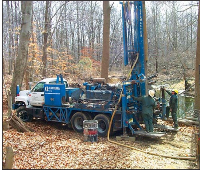
Drilling underway at the Galaxy Spectron site
