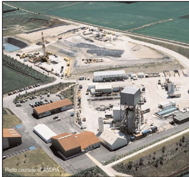
A portion of the surface facilities at Bure during shaft construction.
