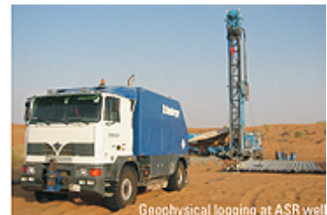
Geophysical logging at ASR well Test drilling at the ASR site.
