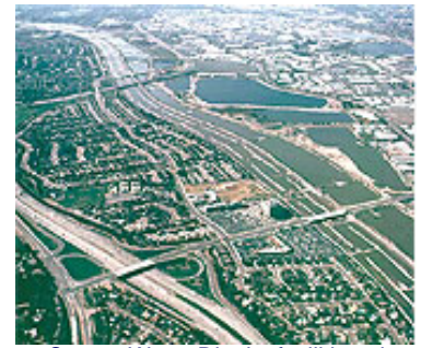
Orange County Water District facilities along the channel of the Santa Ana River
